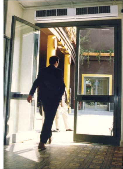
Mounting next to each other to cover different door widths.
