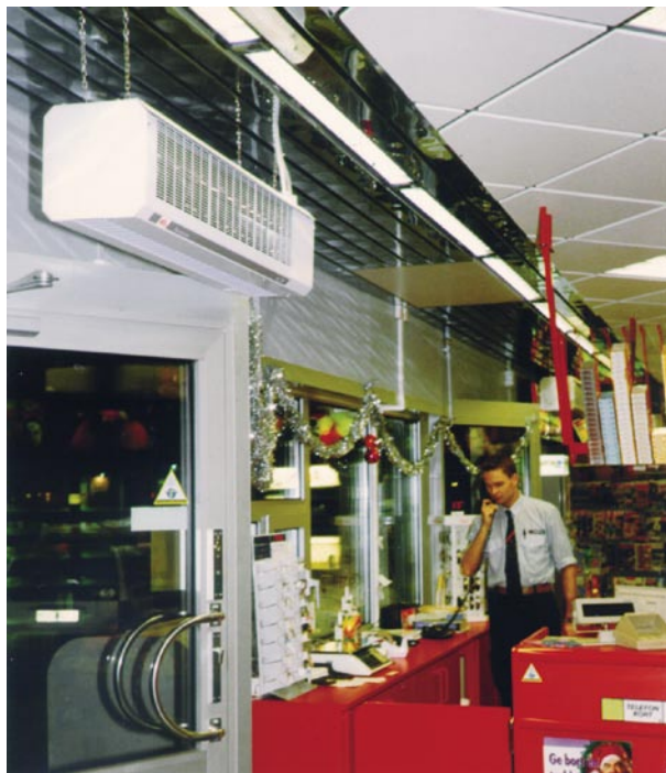
Suspension from the ceiling by drop-rod.
