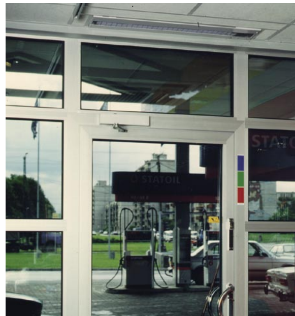
Mounting in a false ceiling
